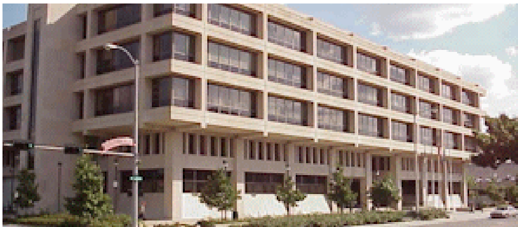
Robert V. Denney Federal Building
